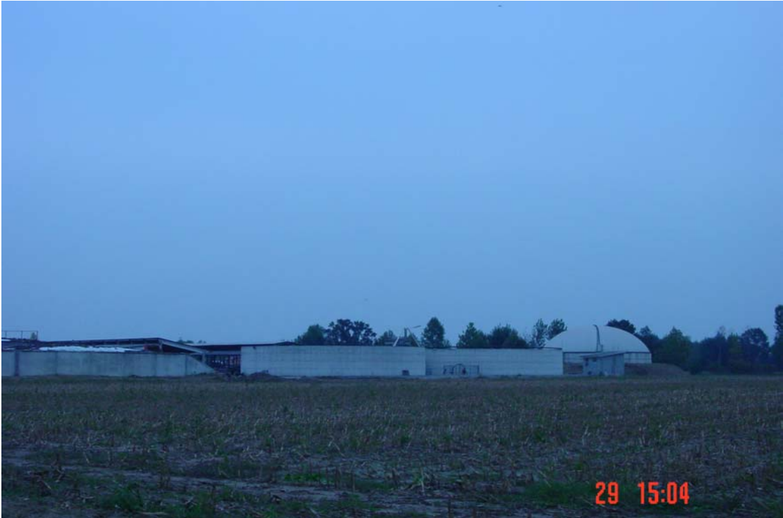
Fosses purins i digestor de gas
